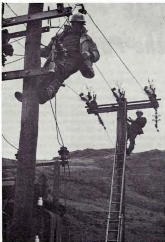
Beginning of the end for Line One. Linesman, W. Pritchard (left) and chargehand linesman Andrew Easton (right) set about removing the conductors.
