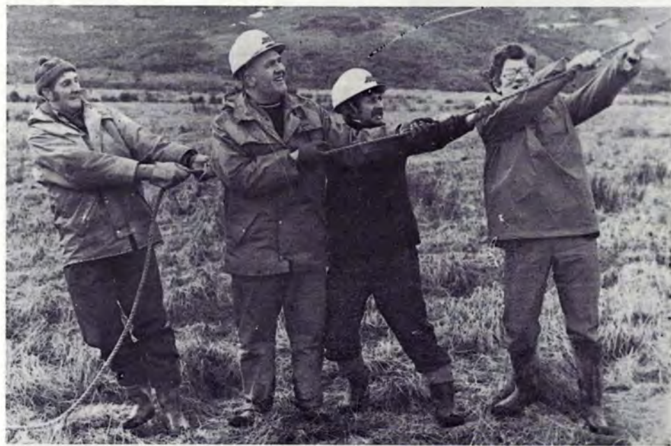
Putting their backs into it to raise the line into position. Left to right: Eric Corfield (driver), Arthur Morris (linesman), Ronnie Hughes (linesman) and Keith Herniman (2nd engineer).
