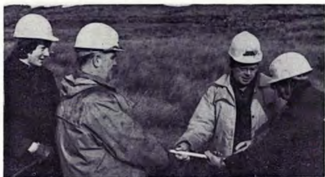
Repairing a broken line with a compression fitting. Left to right: Dyfed Wynne, Arthur Morris, Conway Evans and Ron Hughes.
