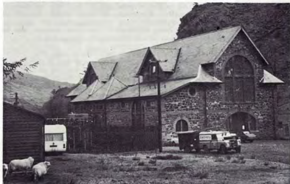
Cwm Dyli power station in its rural setting.
