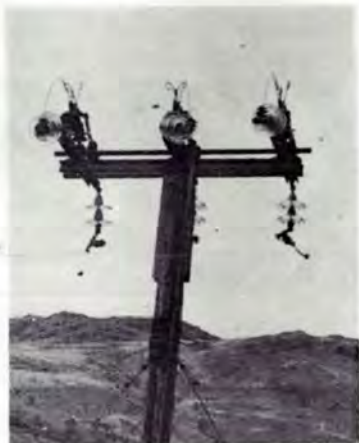
The end of an era—Pole One, Line One, shorn of its conductors.
