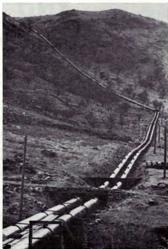
The twin pipes which bring the water power for Cwm Dyli down the mountainside.
